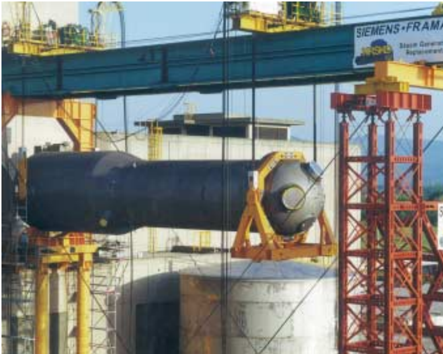
A steam generator on a lifting ring before its installation (May/June 2000).
