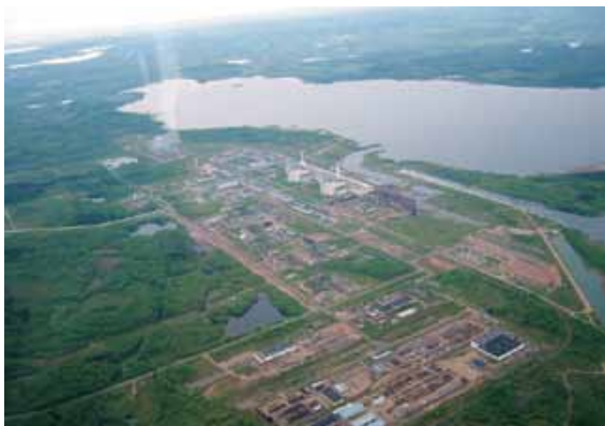
Ignalina NPP heat Power Station (building 119) after dismantling. (Source: www.iae.lt)
